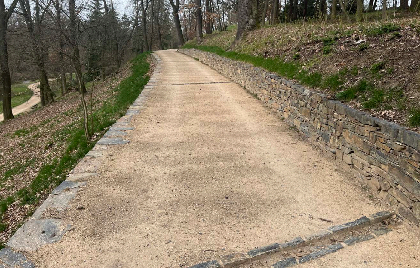
Fig. 11: IROP – road renovation – after completion – Na Mršníku. Source: Jiří Šmída, 2024
