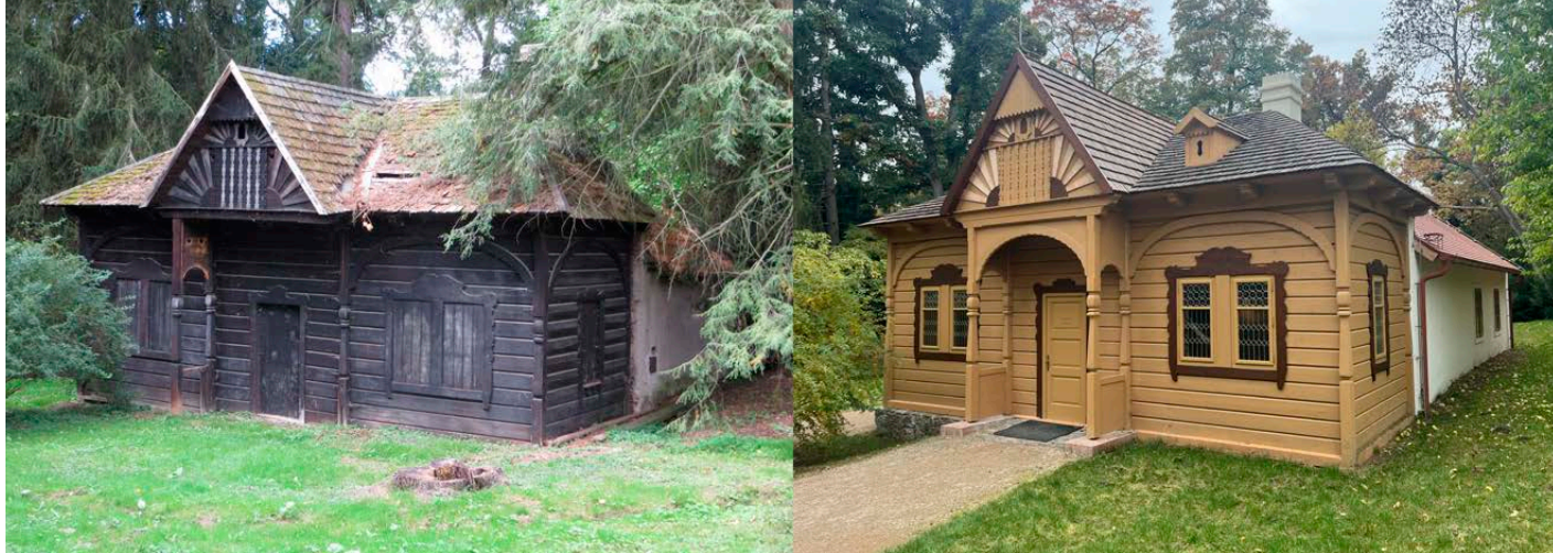
Fig. 12: IROP – renovation of the Former Fish Farm Building. Source: archives of the Průhonice Park Administration, Botanical Institute of the Czech Academy of Sciences
