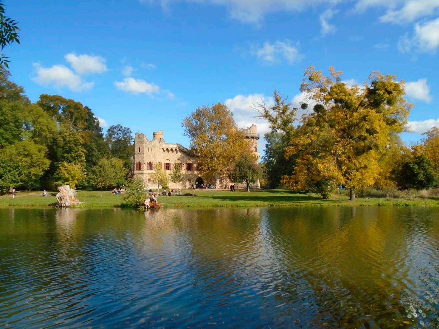
Fig. 12: Janův Castle hunting lodge built in the meander of the Old Dyje River with partially preserved park landscaping in its surroundings. View from the south. Photo: Roman Zámečník, 2023
