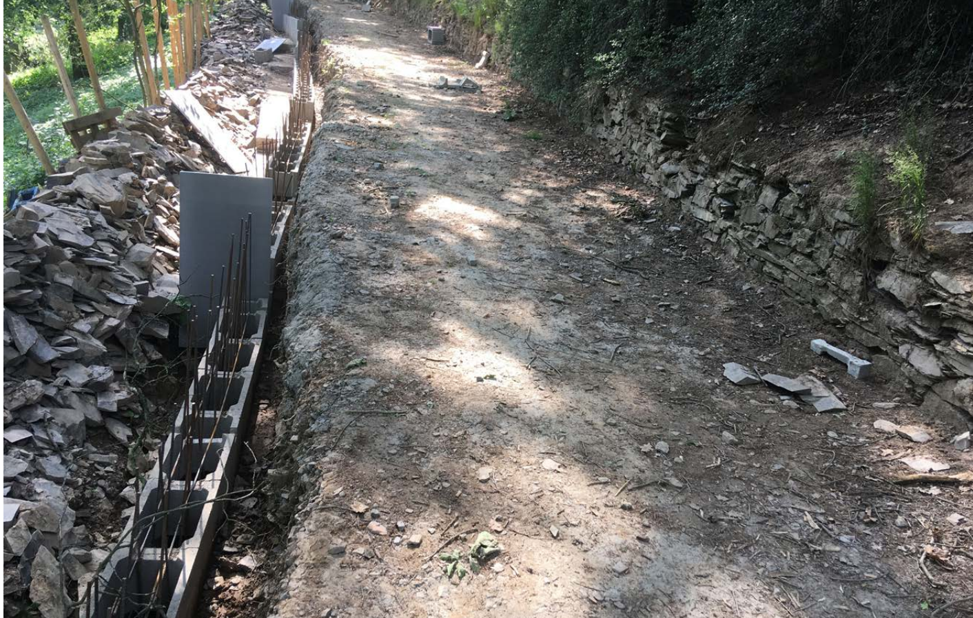
Fig. 10: IROP – road renovation – before implementation – Na Mršníku. Source: Jiří Šmída, 2022
