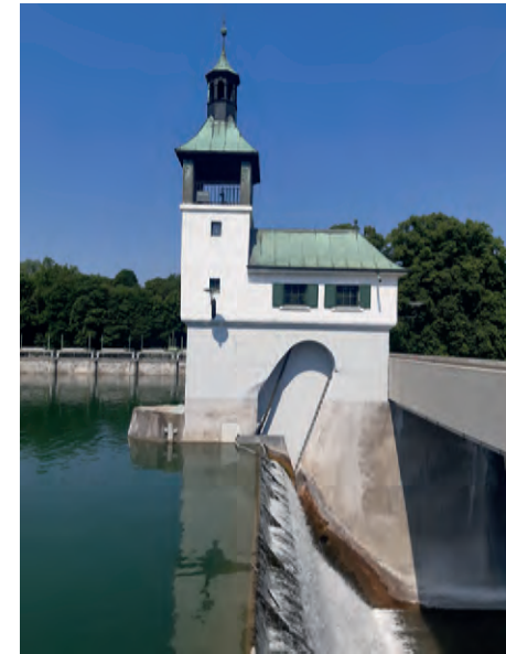
The Hochablass Weir was reerected in concrete in 1910 after a heavy flood had destroyed the older wooden structure. @Alexandra Lotz
