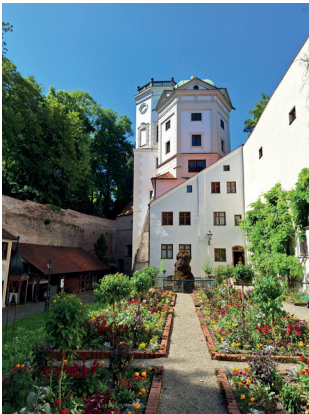
Water Towers at the Red Gate @Alexandra Lotz
