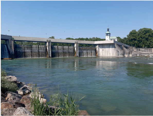
Hochablass Weir at the river Lech @Alexandra Lotz
